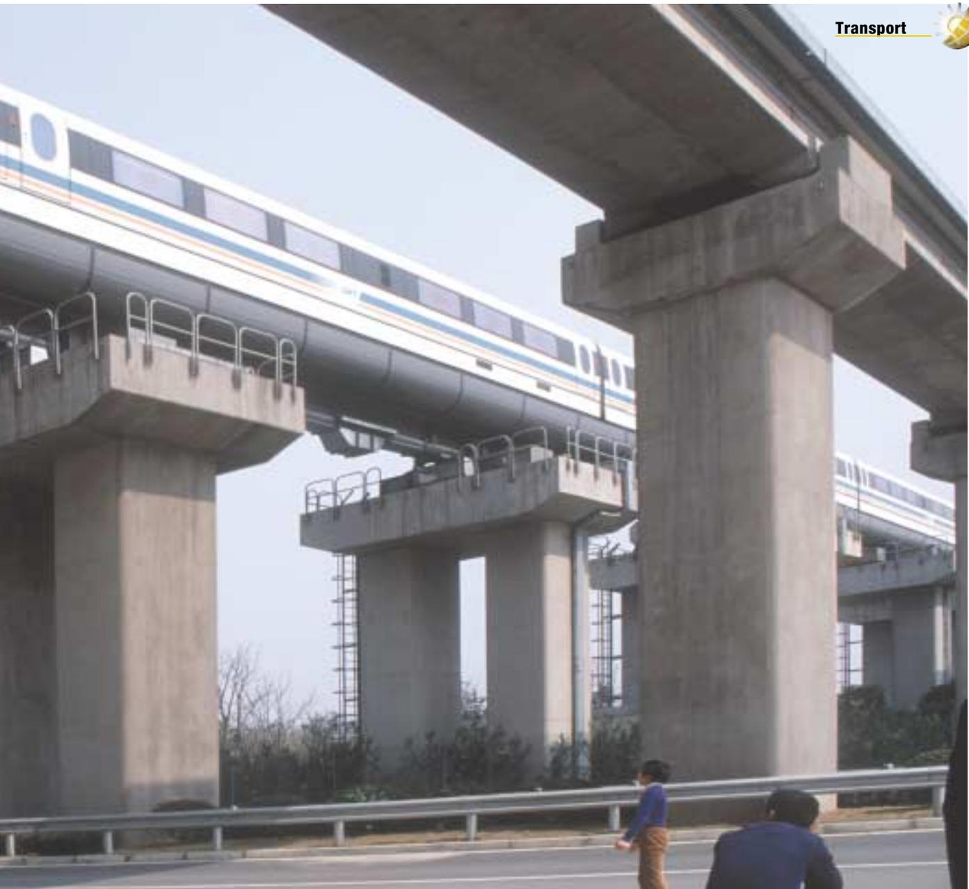
***I-shaped hybrid girders – reinforced-concrete centre girders with steel cantilevers – were chosen to support the guideway as they offered the best rigidity, ride, wear, noise, cost, handling and heat expansion characteristics.***
